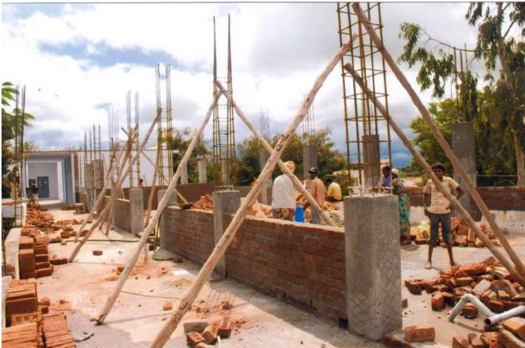
Construction of Additional Classrooms
